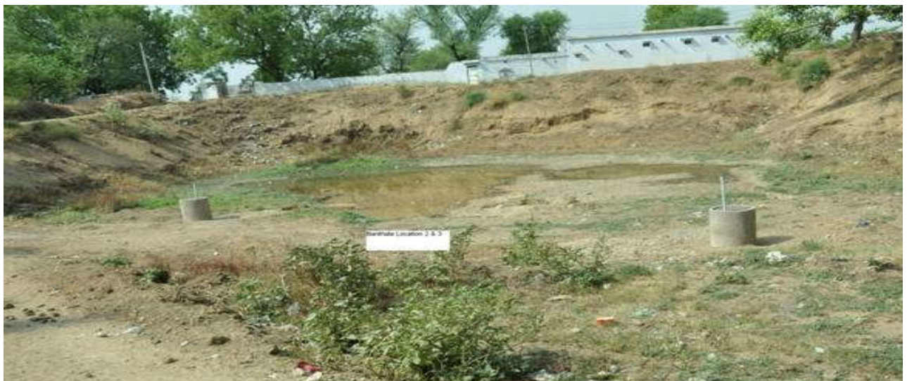
Photograph of water bodies with recharge shafts were taken before rains, after rains on 25.8.12 when the water bodies had received rain water and after seven days on 2.9.12. Rain water was recharged of full quantity at some locations and partial at some locations where bodies were of bigger size. Dosod Low Land Shaft near CGWB
