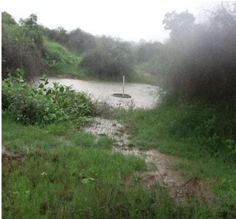
Recharge Shaft Status on 25.8.12 after Rains
